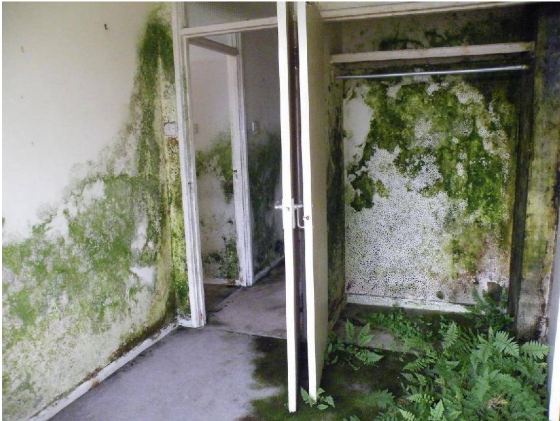
Appendix 2j: Wilton, Thornton Crescent, SP2 0BF - 2009 – units released by the DIO with extensive mould damage and ingrowing plants
